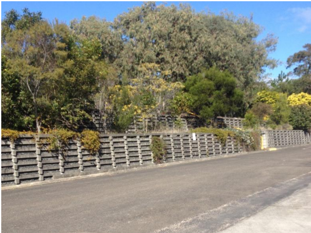
Plate 7.8: Mannering retaining wall below main carpark
