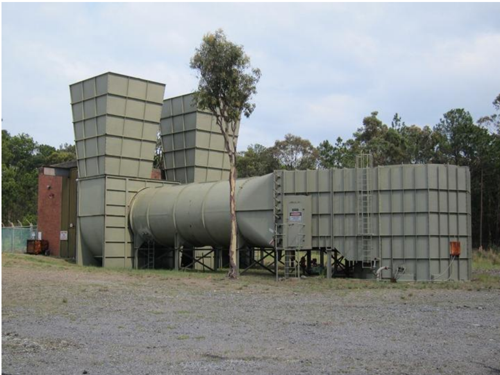
Plate 7.6: Mannering main ventilation fans
